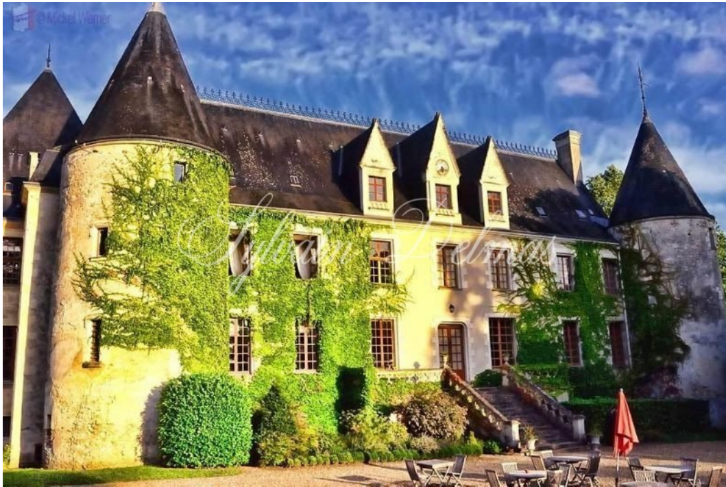
REIGNAC-SUR-INDRE, Indre-et-Loire, FRANCE
